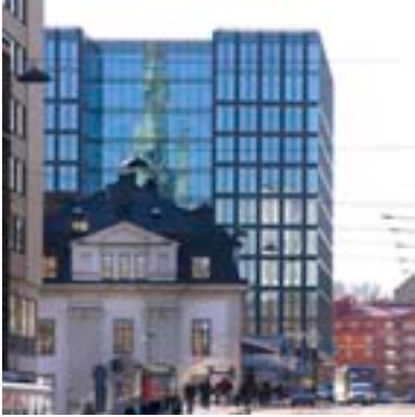
Centralstation and Stockholm Waterfront. Source: White Arkitekter AB, Jarl Asset Management AB
