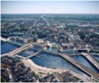
Aerial view of the draft plan for a new Slussen. Source: City of Stockholm / Foster+Partners and Berg Arkitektkontor AB
